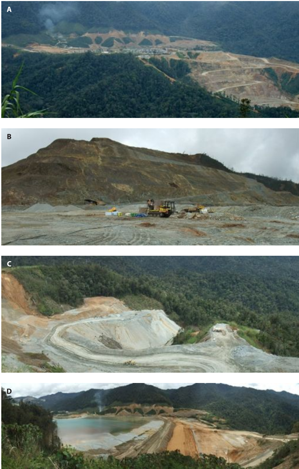
FIG 10 – The Hidden Valley mine complex, April 2012: (A) view from the mine camp showing the process plant in the centre, Hamata open cut on the right and mountains in the background; (B) Hidden Valley mine showing acid mine drainage on mine wall; (C) waste rock dump encapsulating sulfidic material to reduce acid mine drainage risks; (D) tailings dam panorama (photos: Mineral Policy Institute, April 2012).
