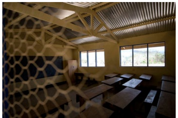
A newly renovated classroom, Kayelekera primary school
