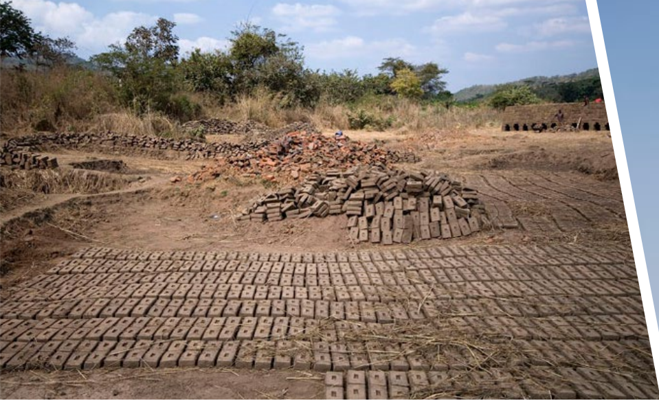
Bricks being manufactured for the primary school, Kayelekera
